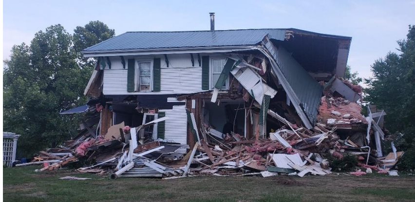
Description of 2 Images: Aftermath of farmhouse destruction
